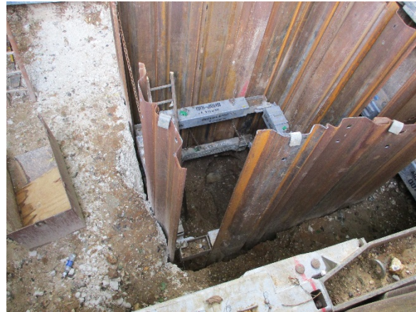
Figure 2: A 5½ meter deep £78k trial hole
