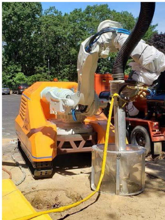
Figure 19 - Excavation operation using the robotic arm
