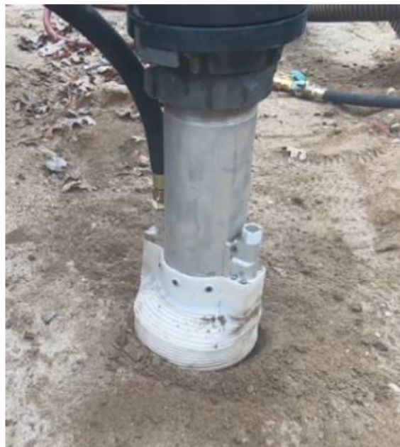
Figure 12 - Excavation Head Cover
