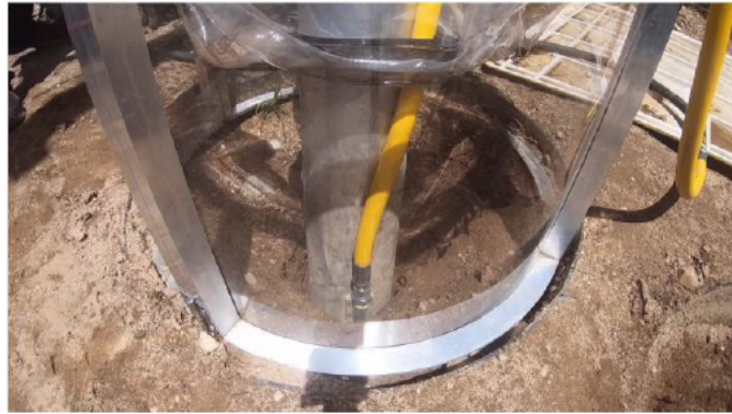
Figure 15 - Excavator head used during manual operation
